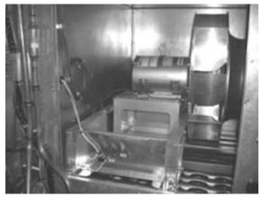
Figure 34 - 11-25 and 30 ton Supply Fan
